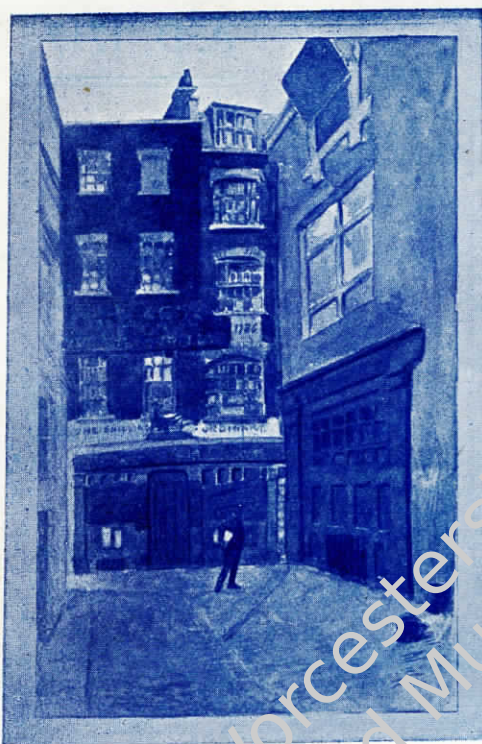
EXTERIOR OF THE "GOOSE AND GRIDIRON", 1896, SHORTLY BEFORE ITS DEMOLITION.
